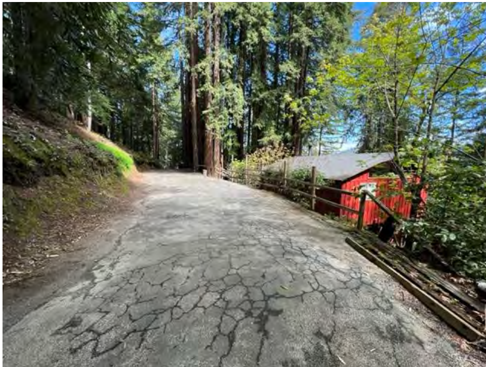
Photograph 16: View looking north along the upper road towards Cabin #10.
