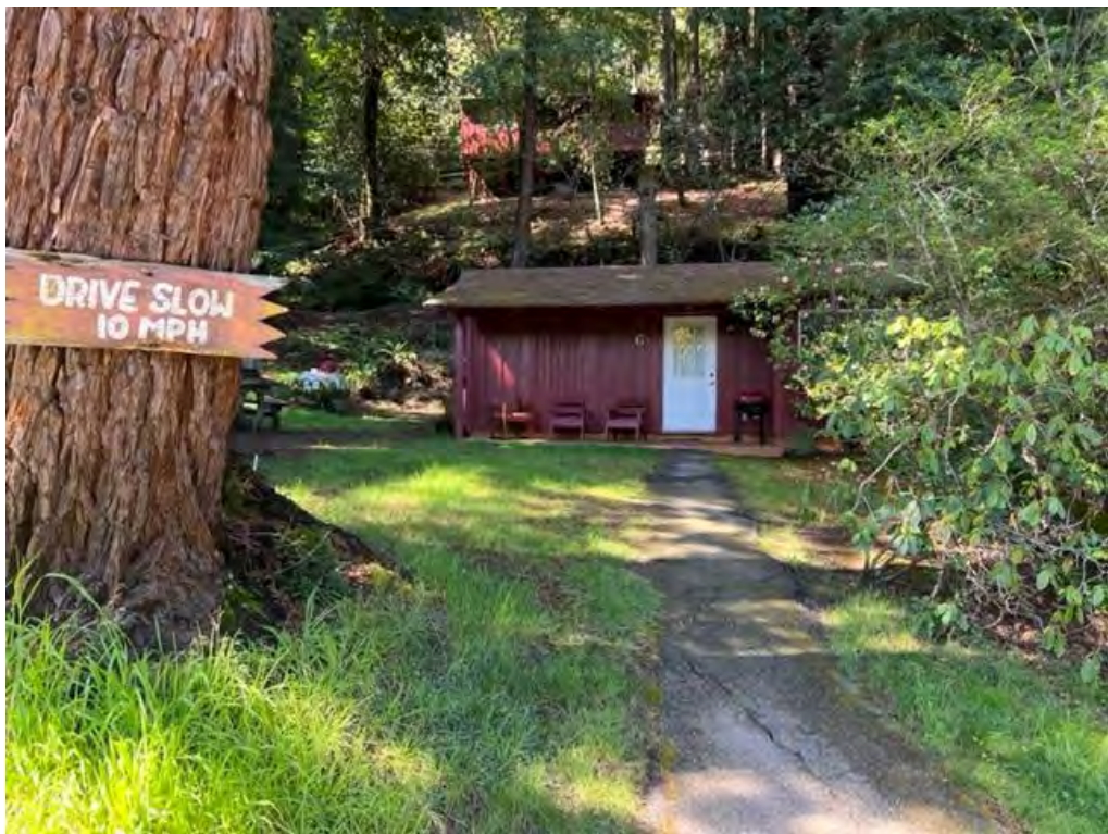
Photograph 6: View looking at Cabin #6.
