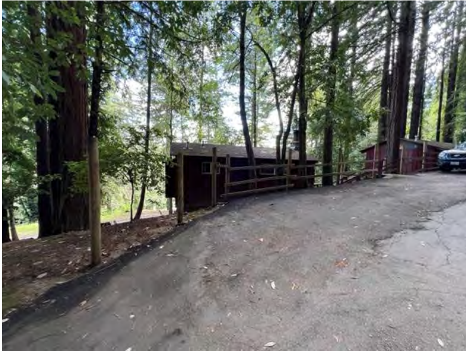
Photograph 11: View looking at Cabin #7.
