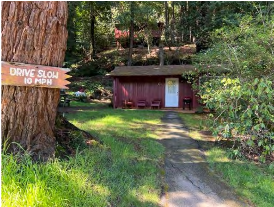
Photograph 6: View looking at Cabin #6.
