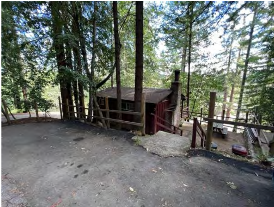
Photograph 12: View looking at the right side of Cabin #7 with the brick chimney.
