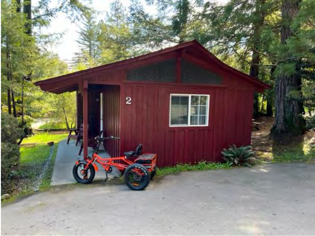
Photograph 9: View looking at Cabin #2.
