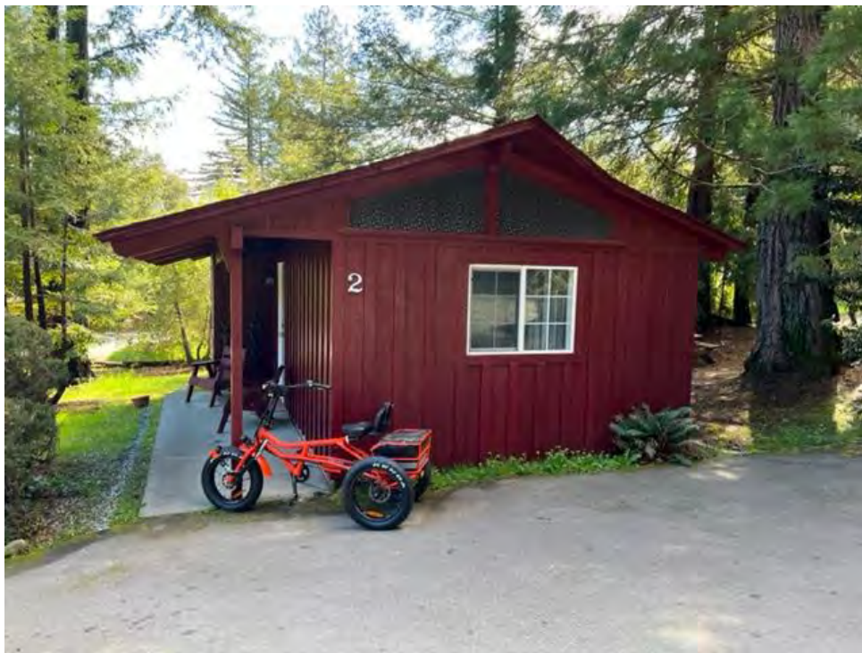
Photograph 9: View looking at Cabin #2.
