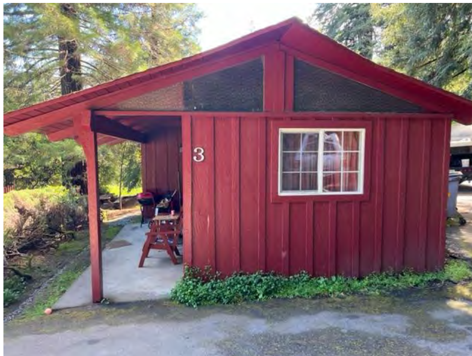
Photograph 8: View looking at Cabin #3.
