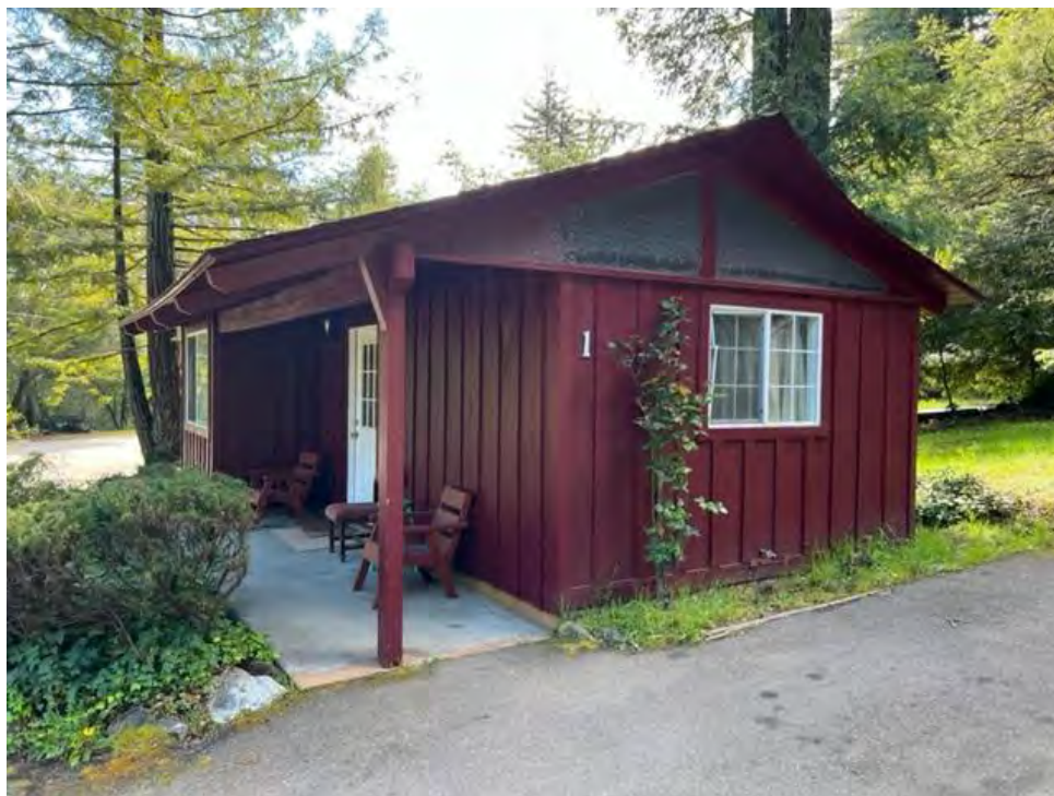
Photograph 10: View looking at Cabin #1.
