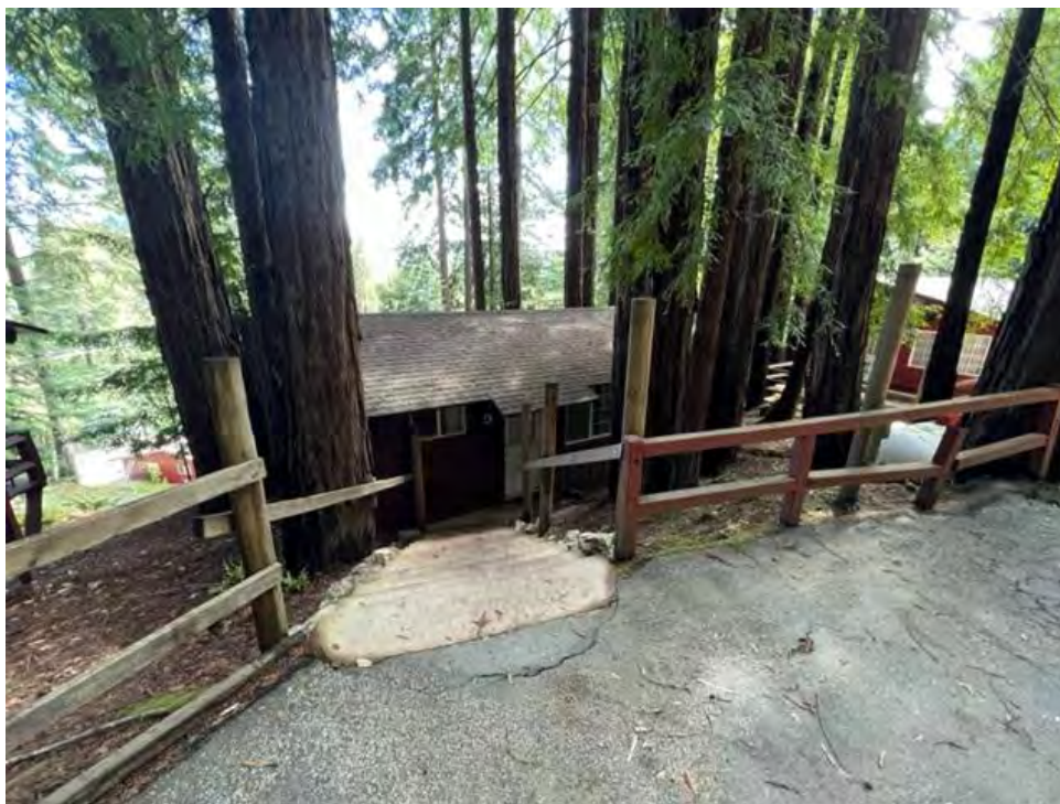
Photograph 14: View looking at Cabin #9.
