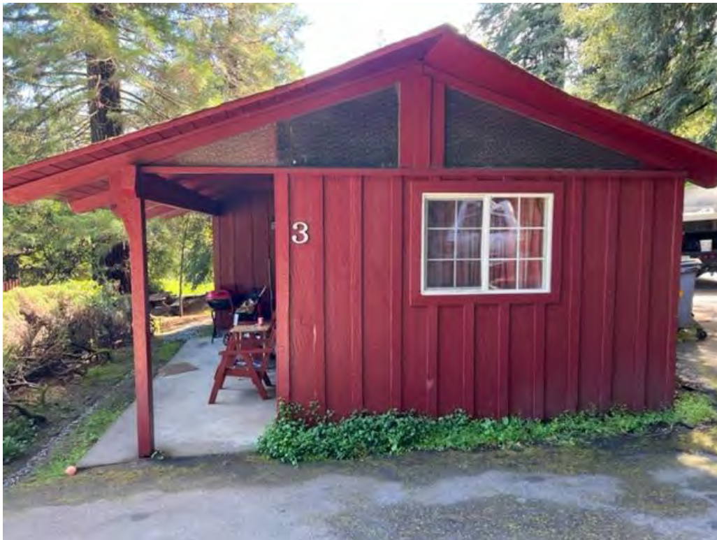
Photograph 8: View looking at Cabin #3.
