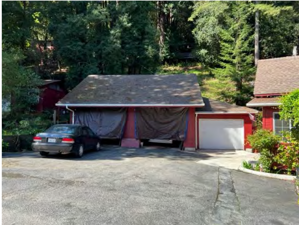
Photograph 4: View looking northwest at the contemporary three-car garage to the left of the manager's office or residence.
