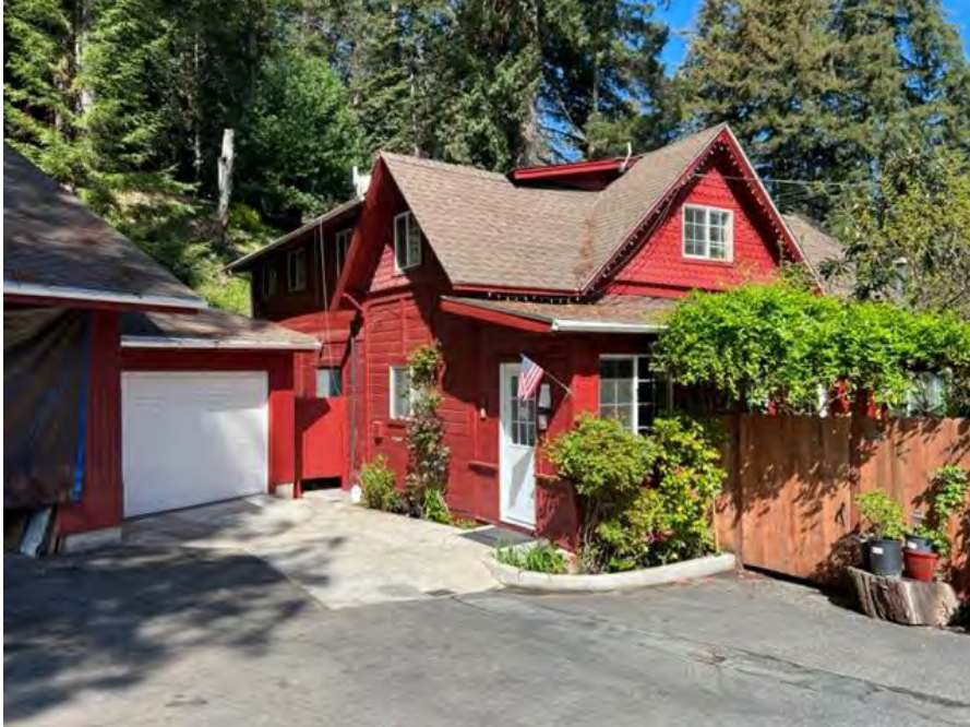
Photograph 1: View looking north at the remodeled manager's office/residence. Note the front porch, once open has been enclosed, a large addition has been added to the rear of the residence, as well as a large three-car garage to the left of the building.
