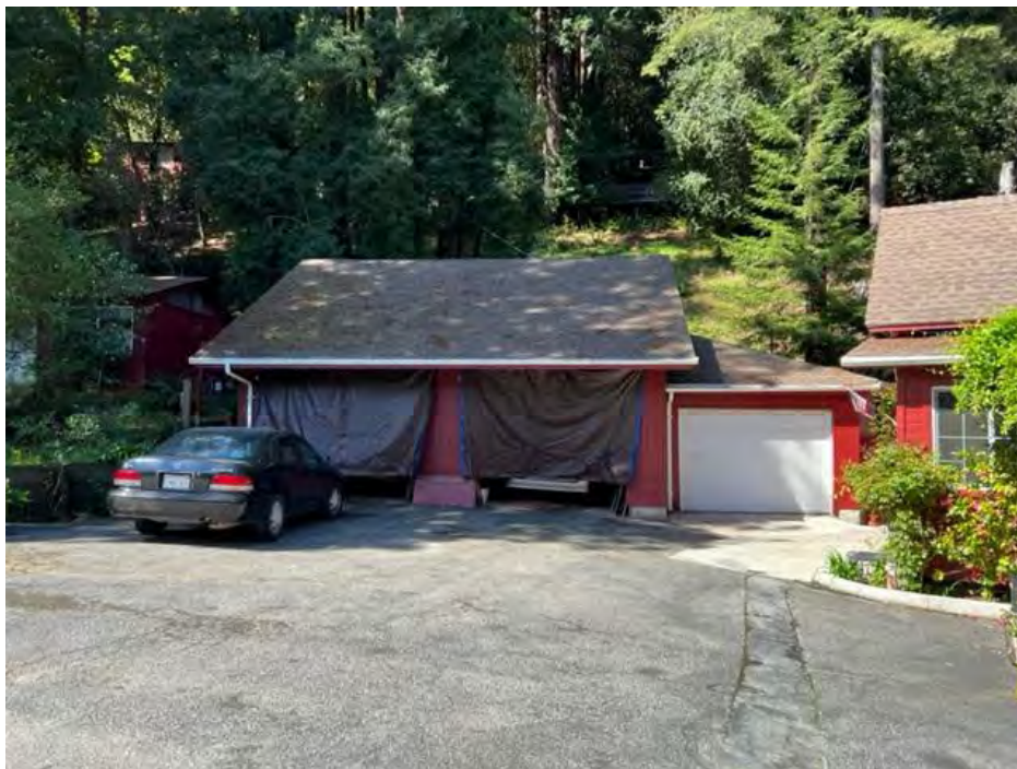
Photograph 4: View looking northwest at the contemporary three-car garage to the left of the manager's office or residence.
