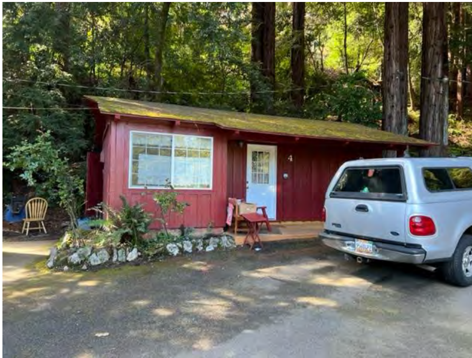
Photograph 7: View looking at Cabin #4.
