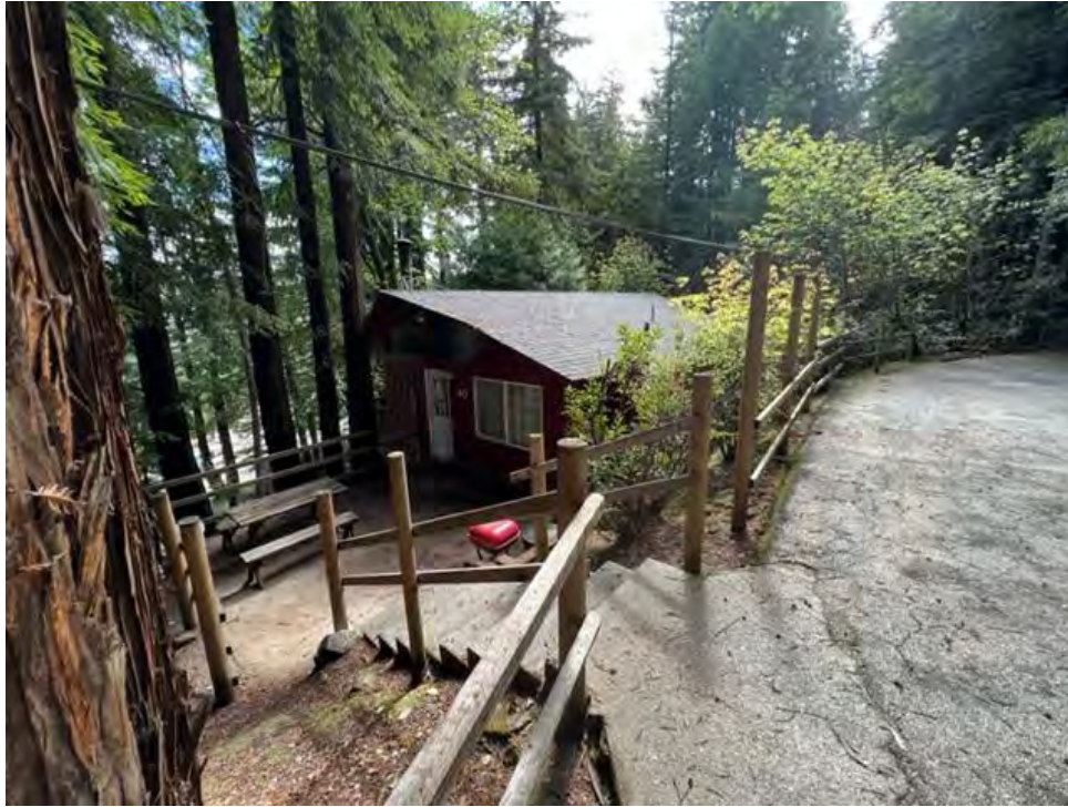
Photograph 15: View looking at Cabin #10.
