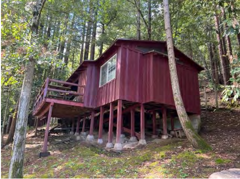
Photograph 17: View of the raised substructure of the upper cabins located on the slope above the lower cabins.
