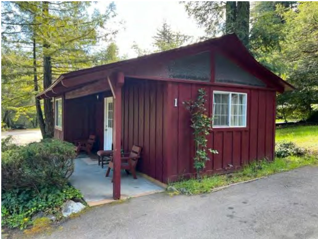
Photograph 10: View looking at Cabin #1.
