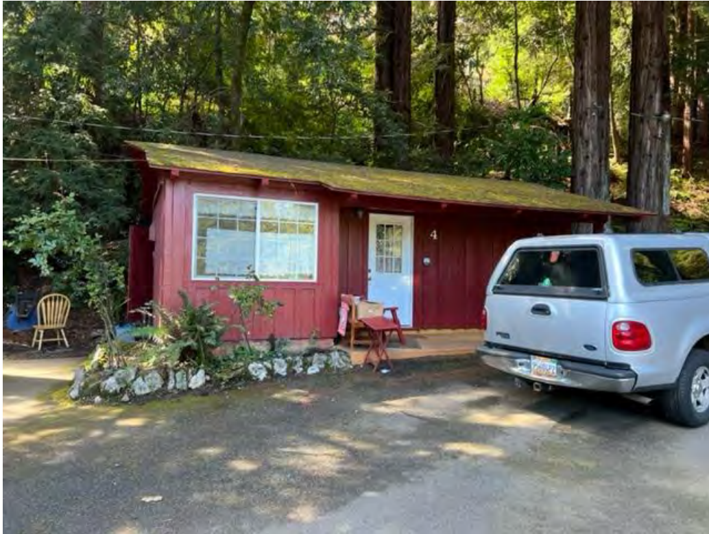
Photograph 7: View looking at Cabin #4.
