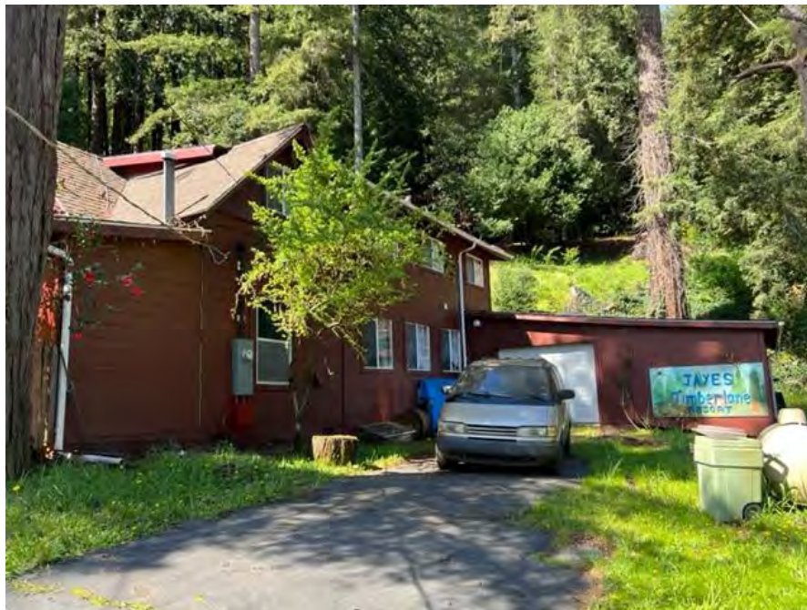
Photograph 2: View looking northwest at the east elevation of the manager's office/residence and the large two-story addition with a shed extension for an additional garage or storage area.
