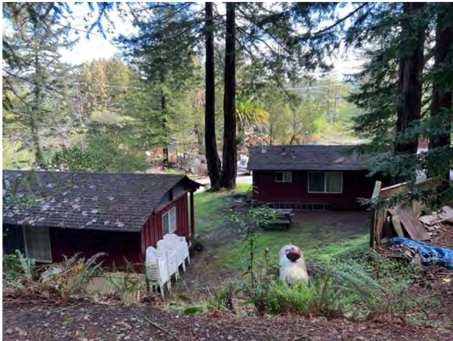
Photograph 18: View looking southwest at the cabins adjacent to the residence/manager's office from the upper road.
