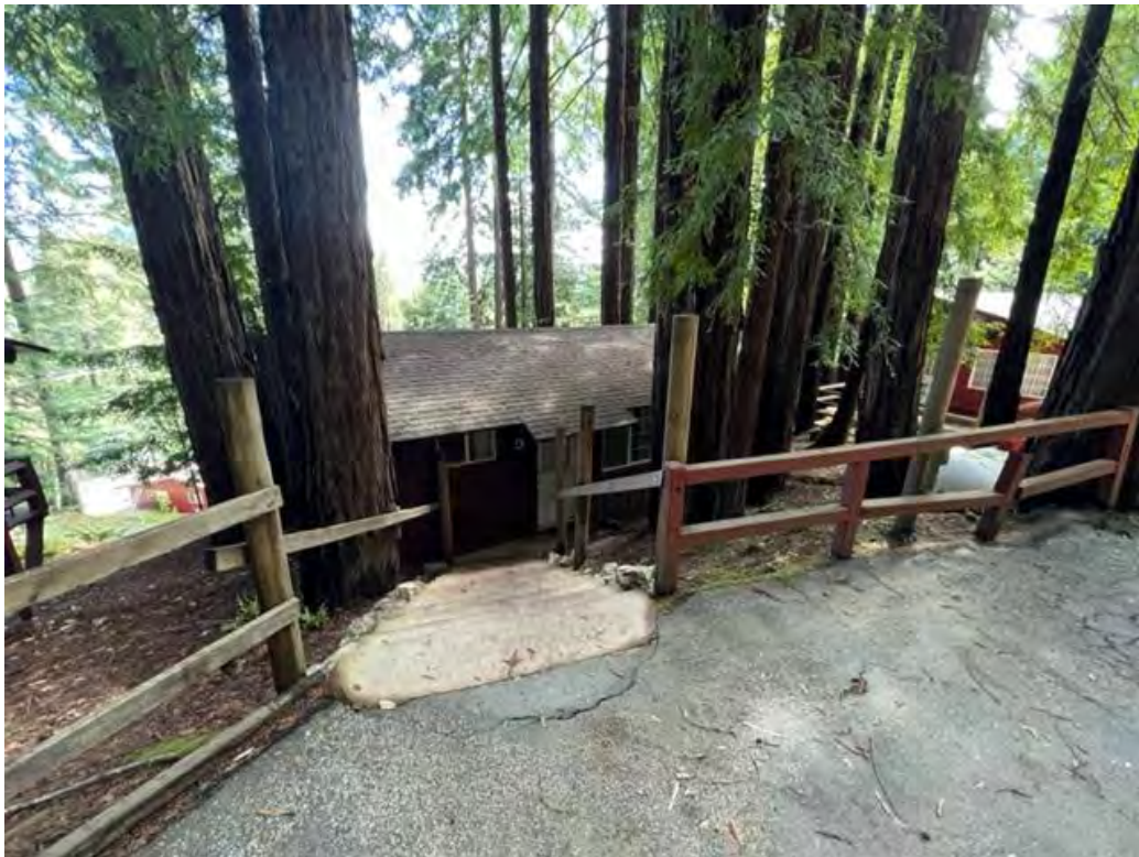
Photograph 14: View looking at Cabin #9.
